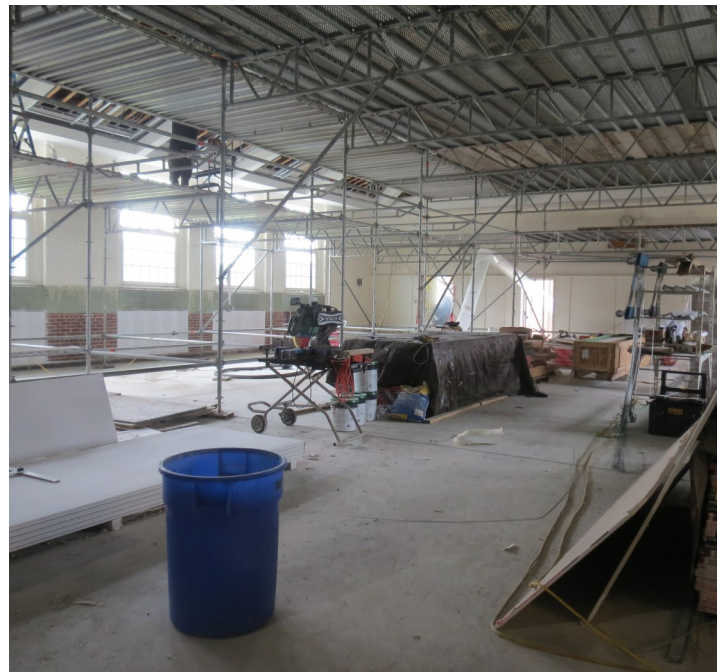
The cafeteria is also under construction.
